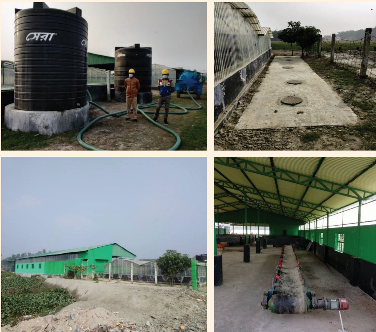
Figure 2 Field visit at fecal sludge treatment plant in Jamalpur Municipality
